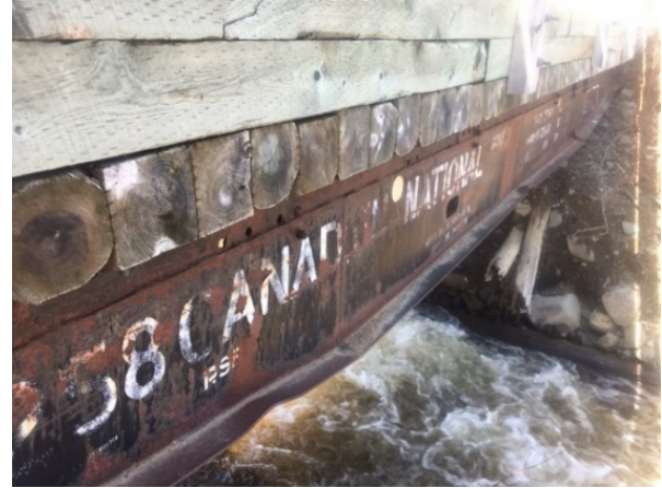
Figure 12: Deteriorated Abutment
