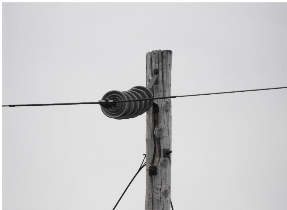
Figure 9: Pole Top with Significant Rot
