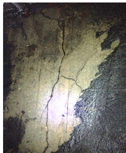
Figure 2: Deteriorated Foundation
