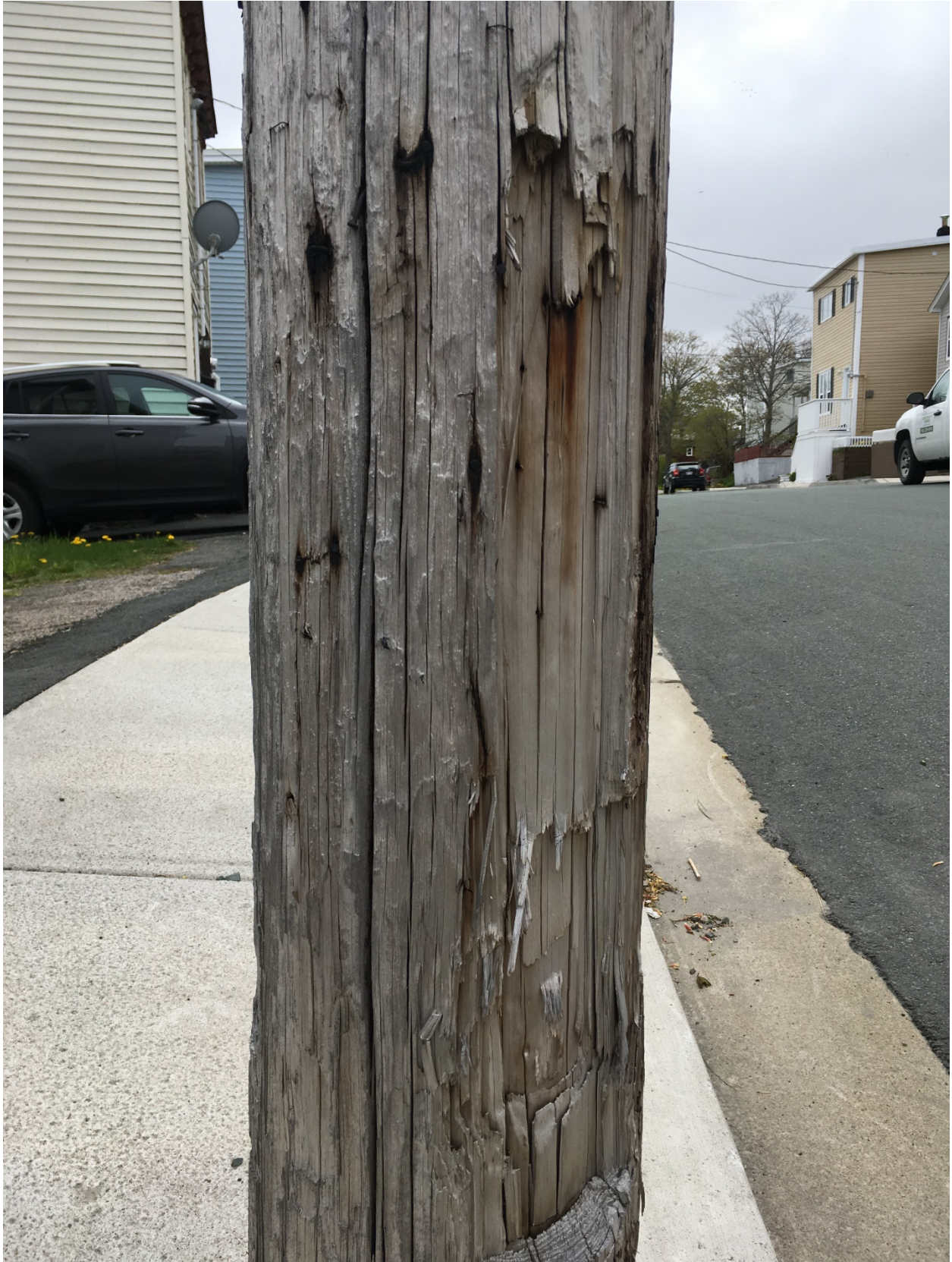
Figure 3 – Deteriorated pole with vehicular damage
