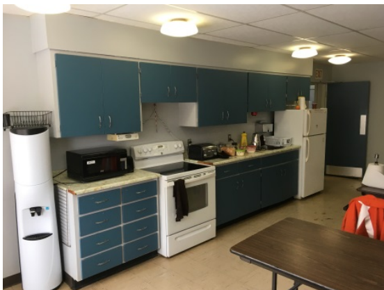
Figure 9: Incandescent Kitchen Fixtures
