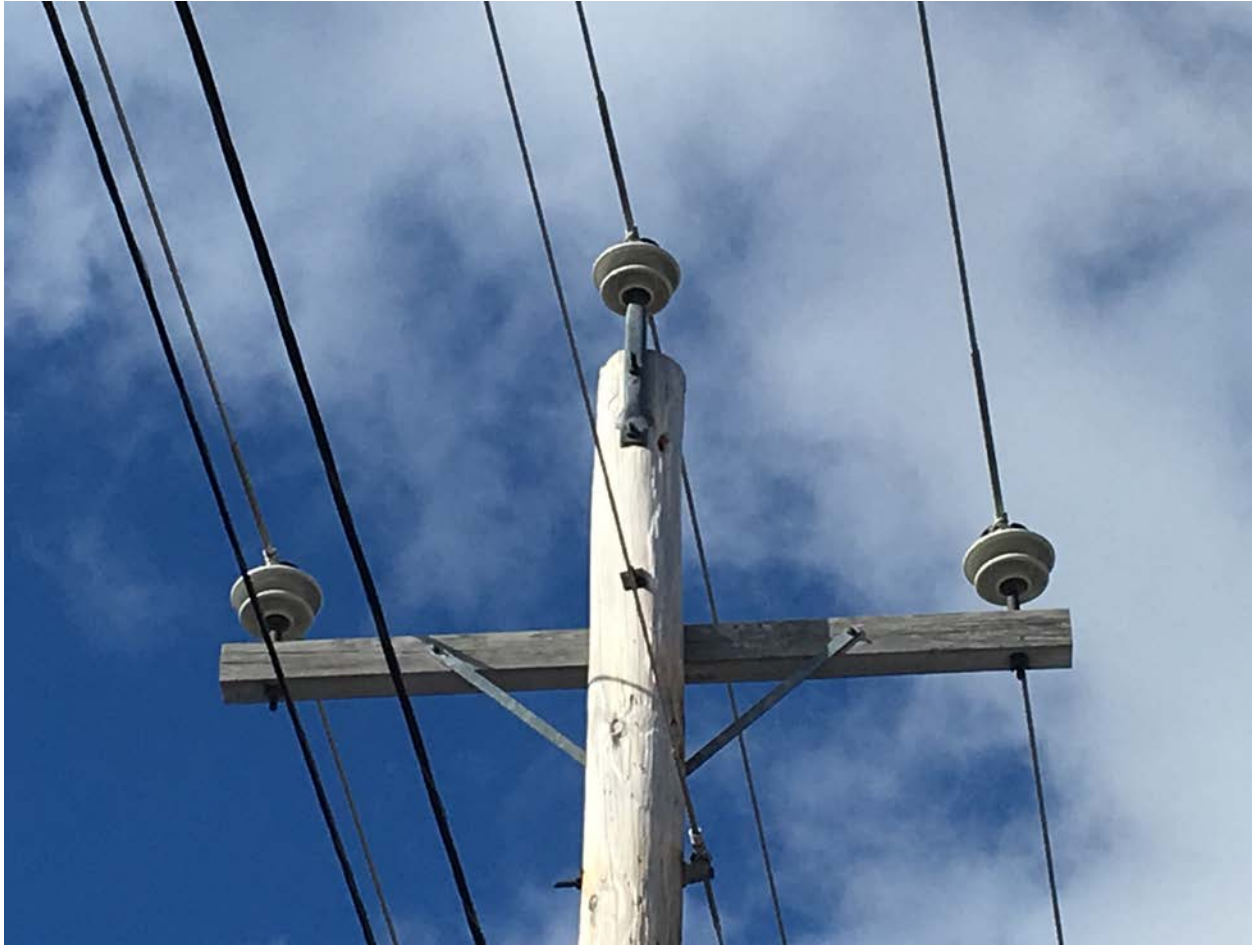
Figure 4 – Two piece insulators
