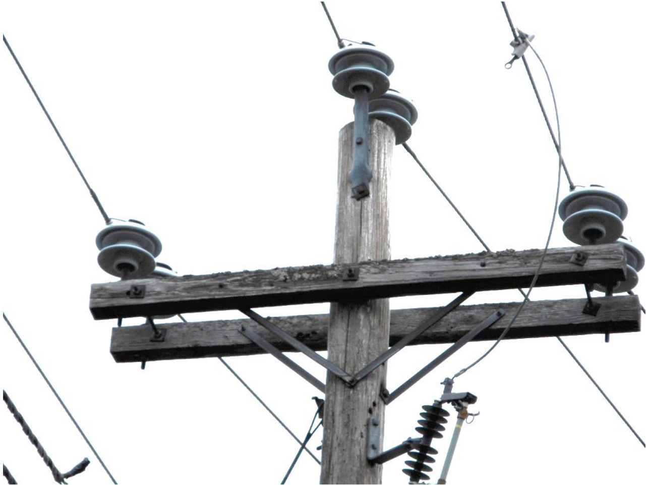
Figure 5 – Two piece insulators and deteriorated crossarm
