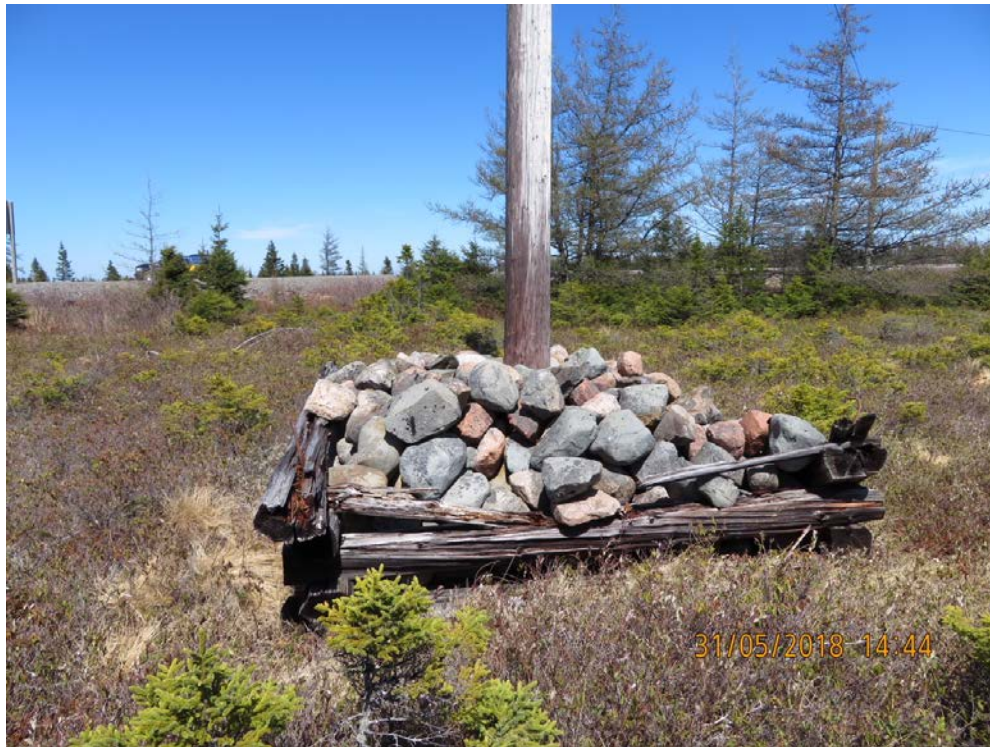
Figure 3: Deteriorated Pole Crib Timber
