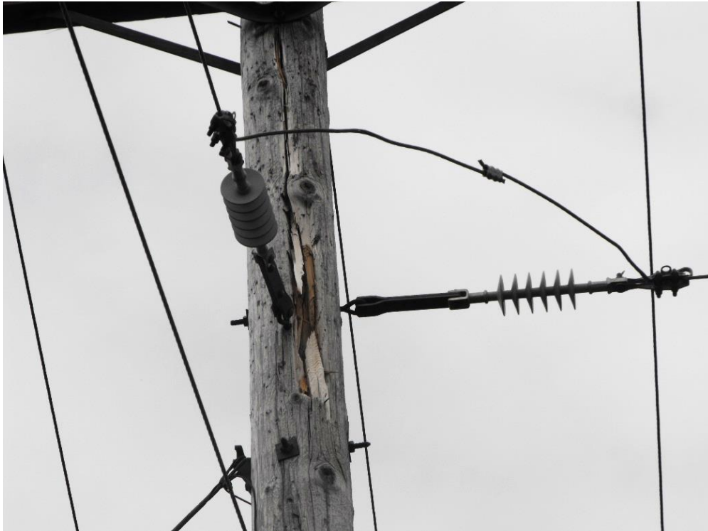
Figure 10: Delamination near Pole Top
