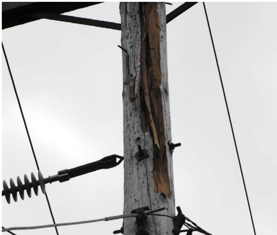
Figure 11: Delamination at Pole Top
