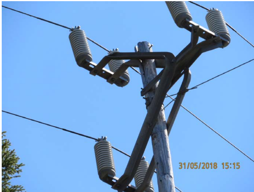
Figure 5: Deteriorated Pole
