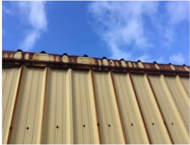
Figure 11: Deteriorated Roof and Eaves
