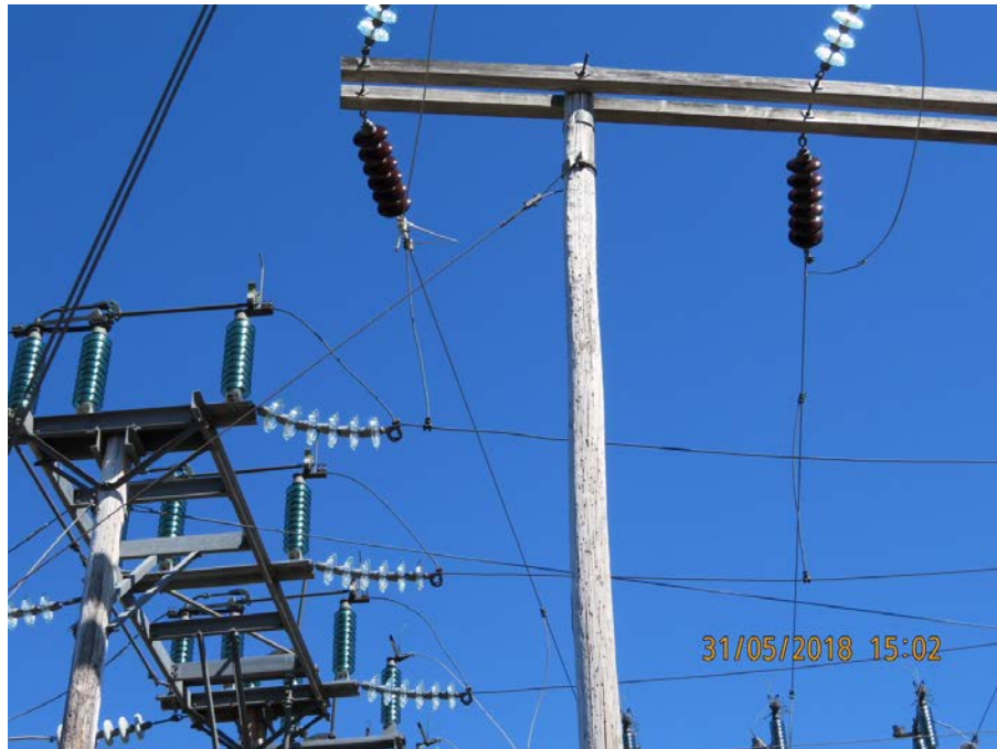
Figure 9: Deteriorated Pole with Vintage Insulators and Connectors
