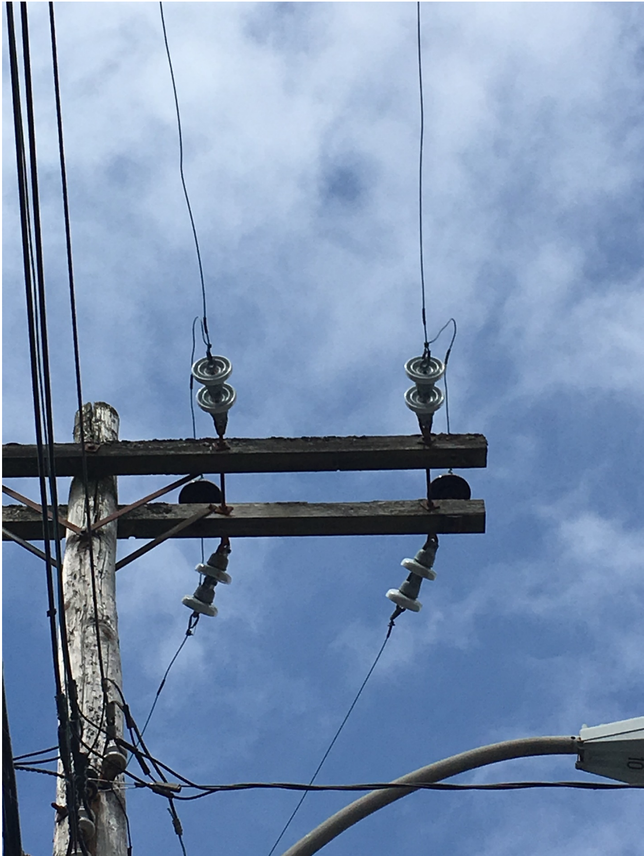
Figure 6 – #6 CU Conductor, deteriorated pole top and 2-piece Insulators
