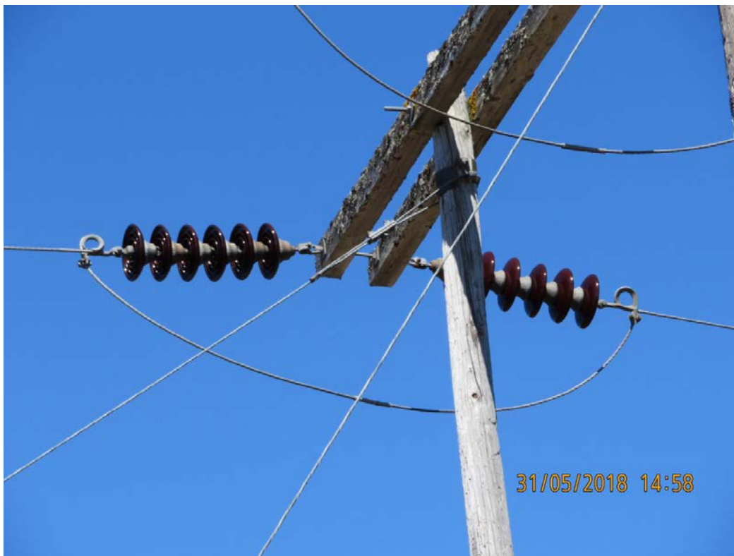
Figure 8: Cross Arm Deterioration
