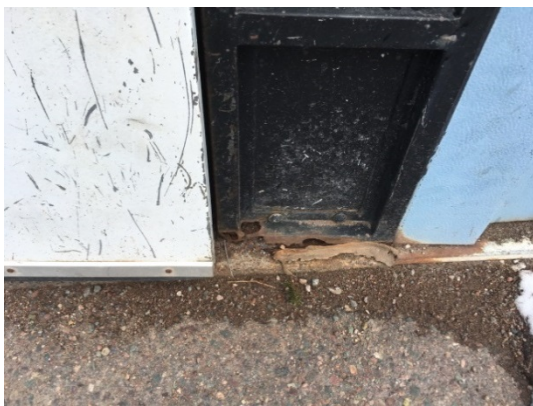
Figure 7: Corroded Door Assembly
