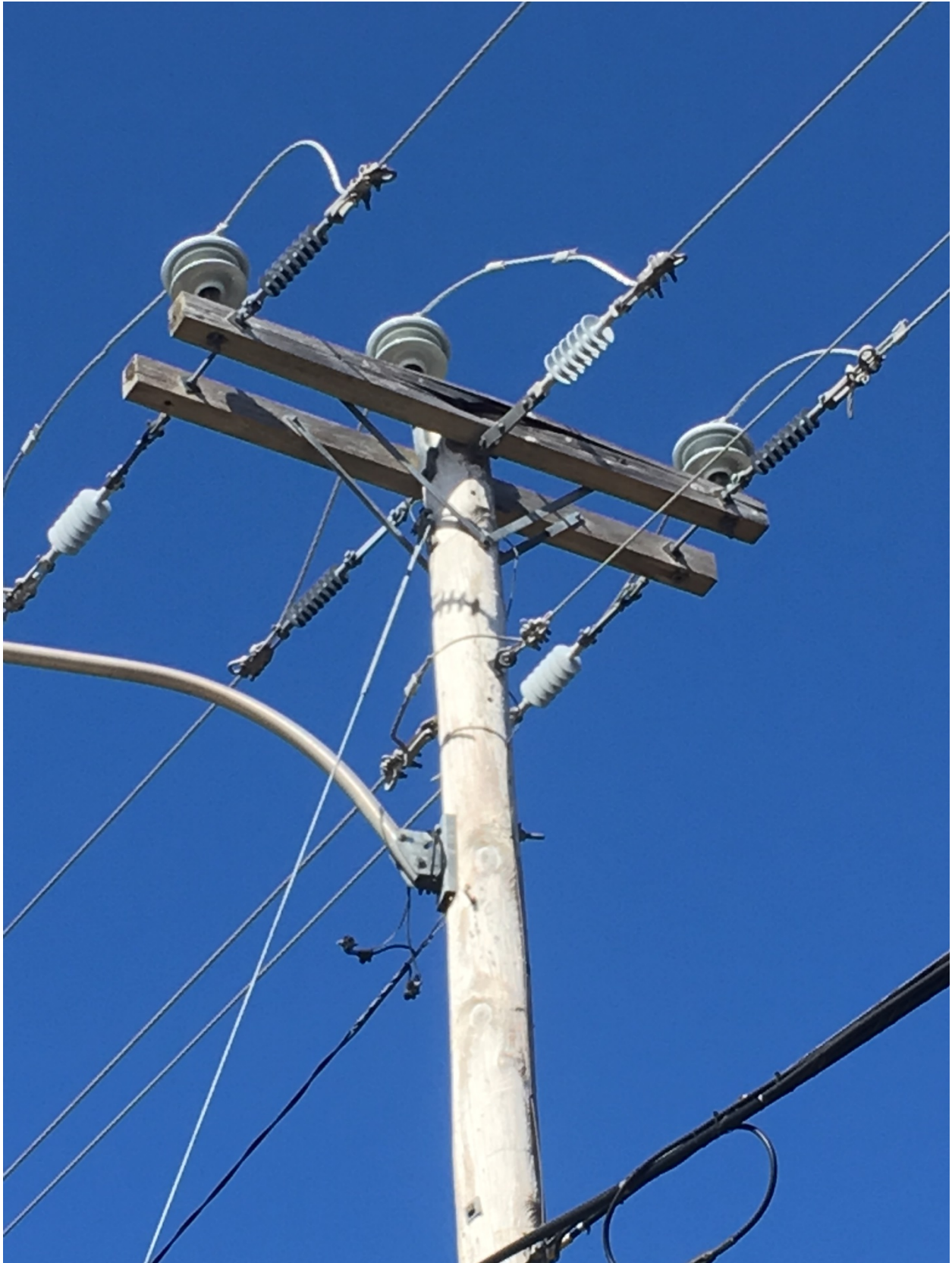
Figure 4 – Deteriorated cross-arm.
