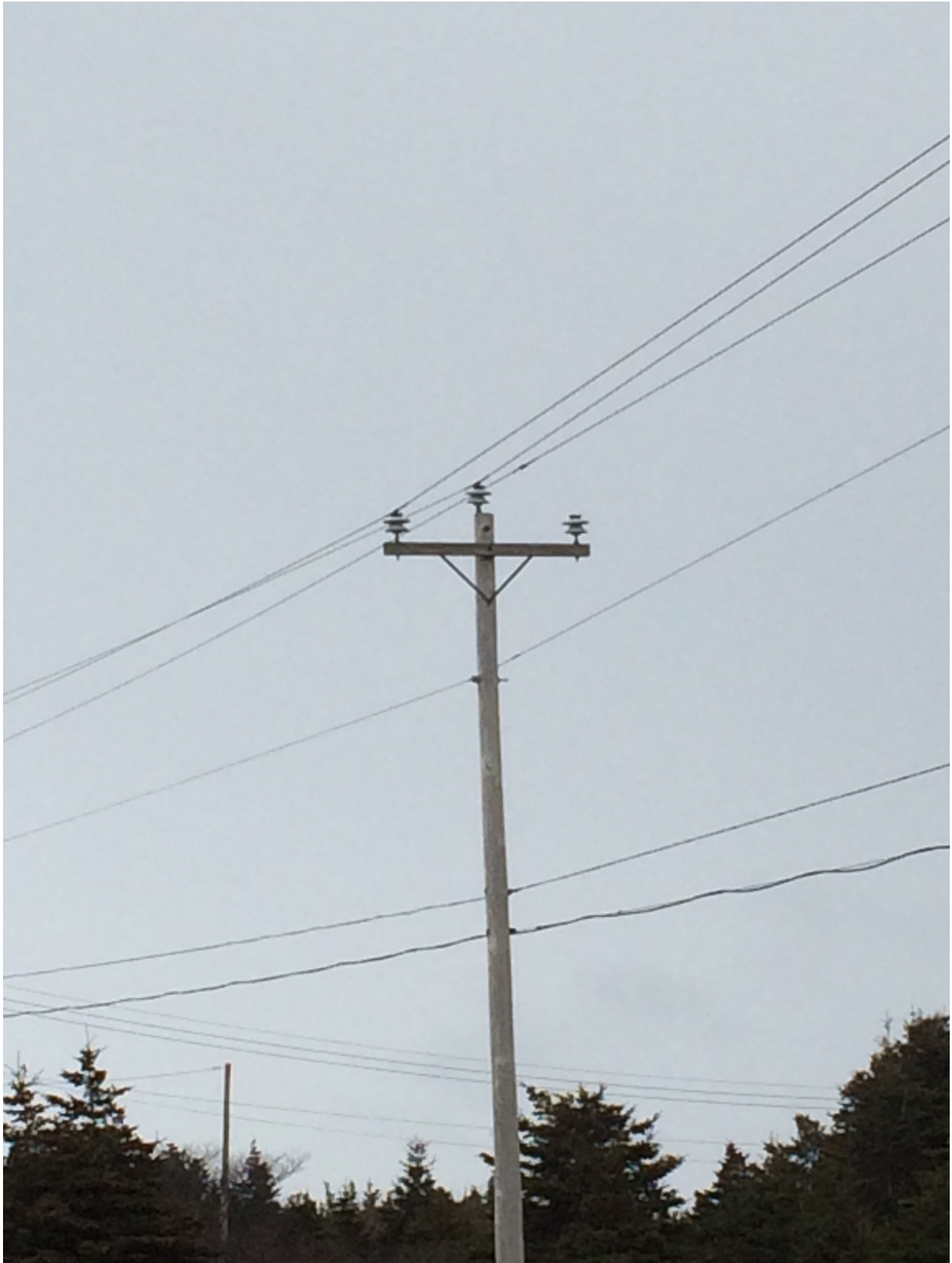
Figure 3 – Floating right side phase caused by broken preform tie.
