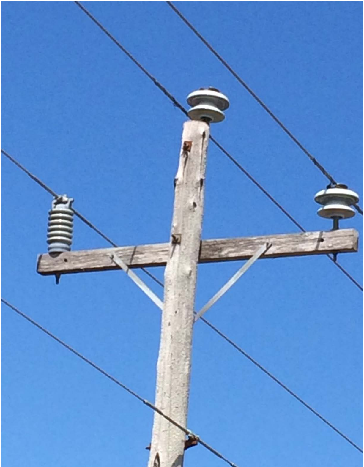
Figure 2 – Floating center phase conductor due to broken preform tie. Note left side insulator replaced
