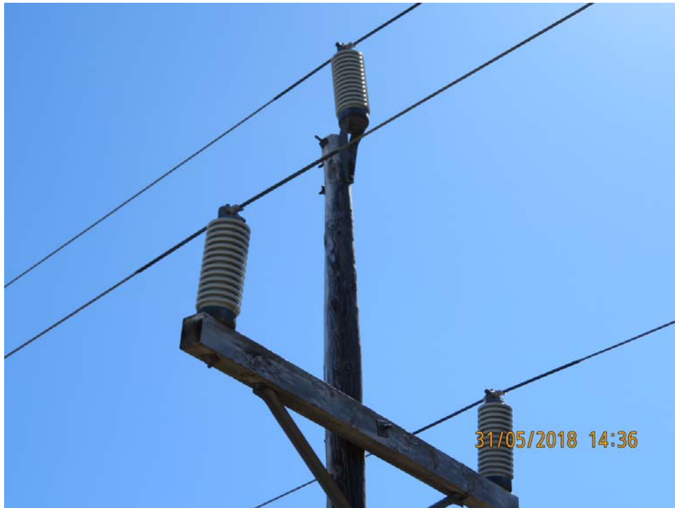
Figure 1: Deteriorated Pole Top
