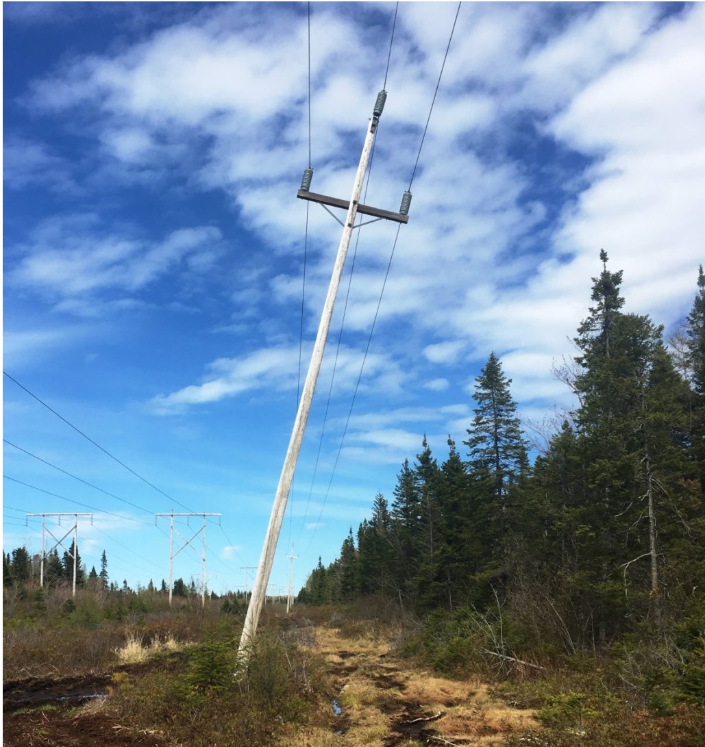
Figure 14: Severely Leaning Structure
