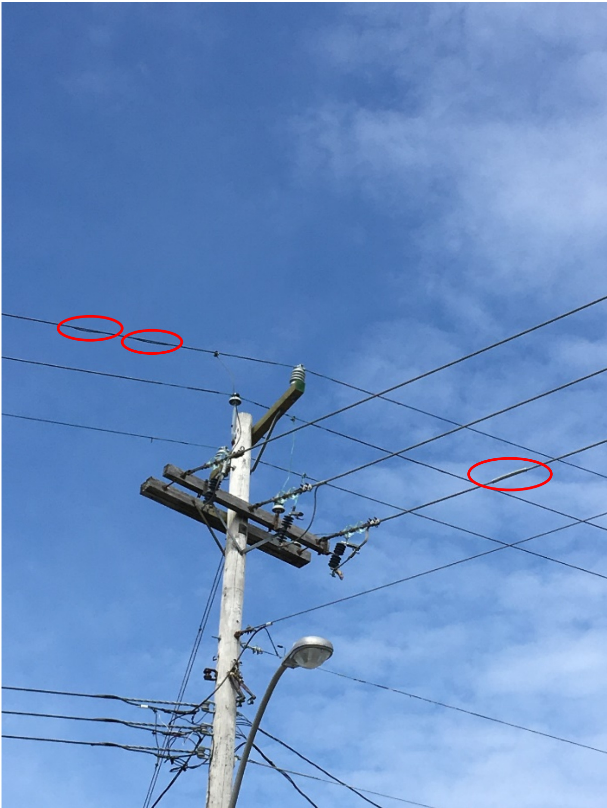
Figure 1 –Sleeved conductor
