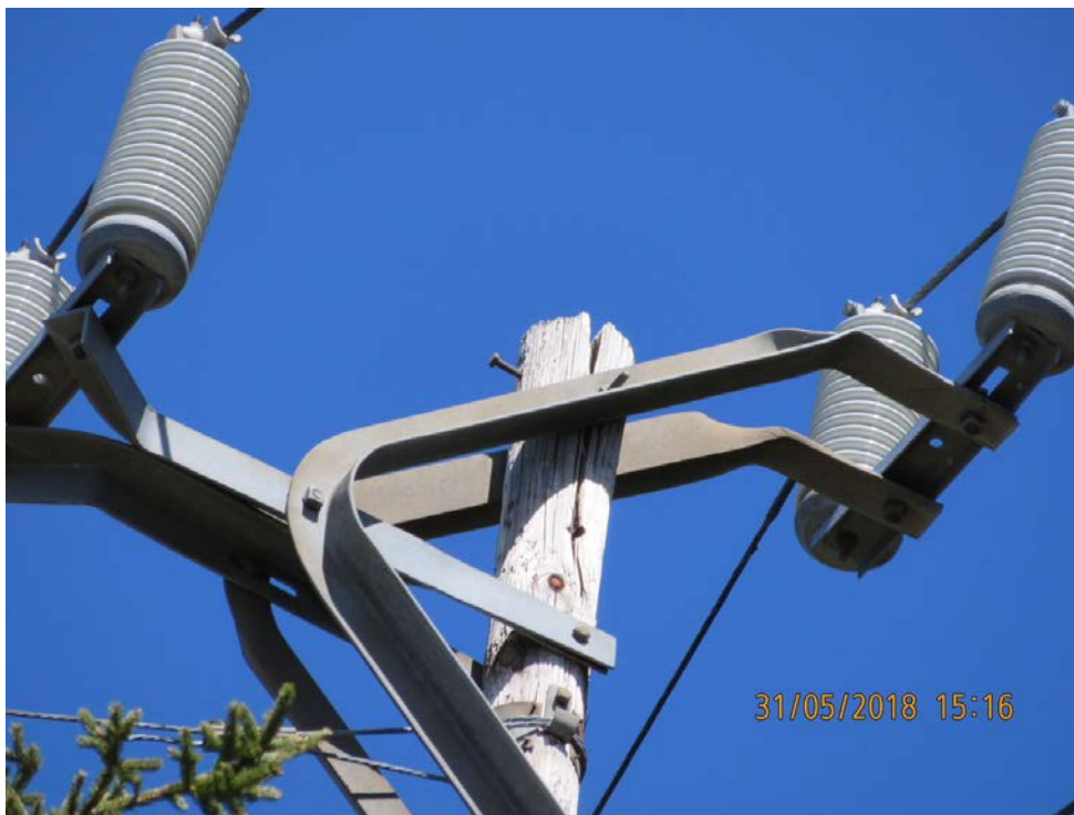
Figure 6: Pole Splitting
