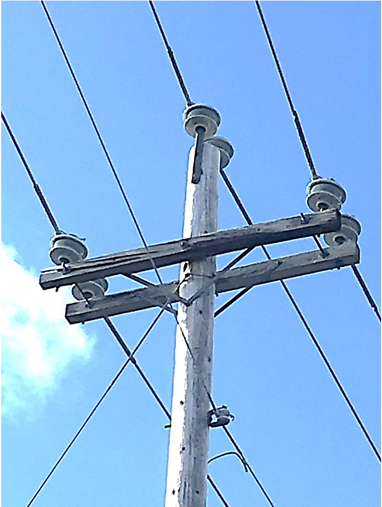
Figure 5 – Split cross-arm on B structure.
