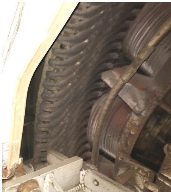
Figure 9: Typical Condition of Generator Stator and Poles
