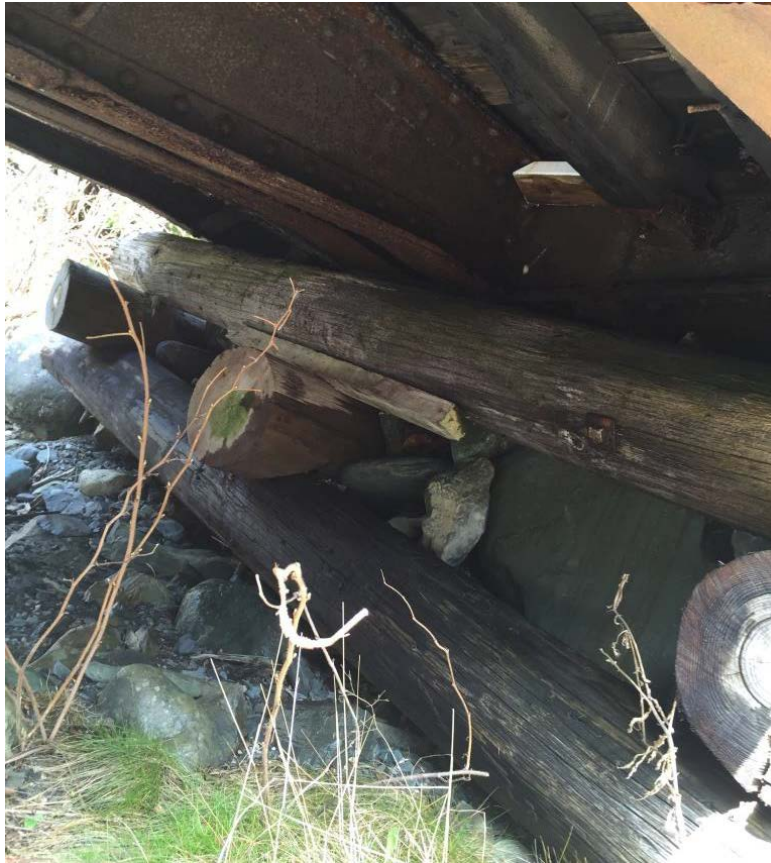
Figure 10: Abutment Deterioration
