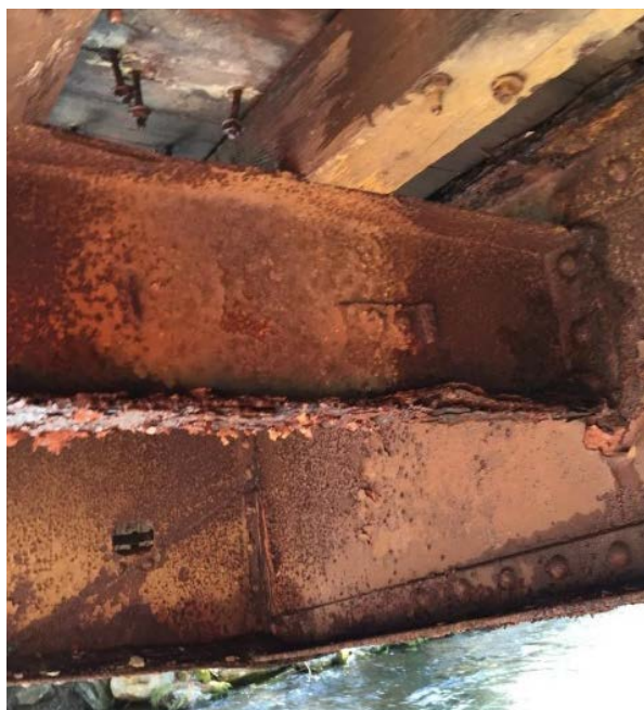
Figure 9: Typical Underside Deterioration
