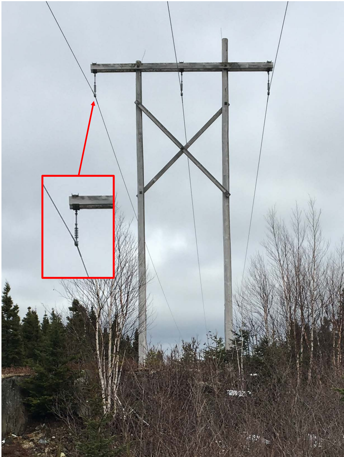
Figure 1 – H-frame transmission type structure with distribution class insulators
