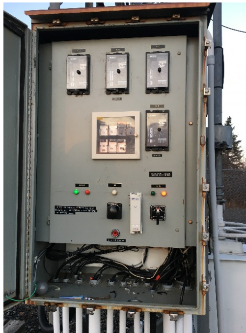
Figure 3: Existing LEW-T1 Protection and Control Cabinet
