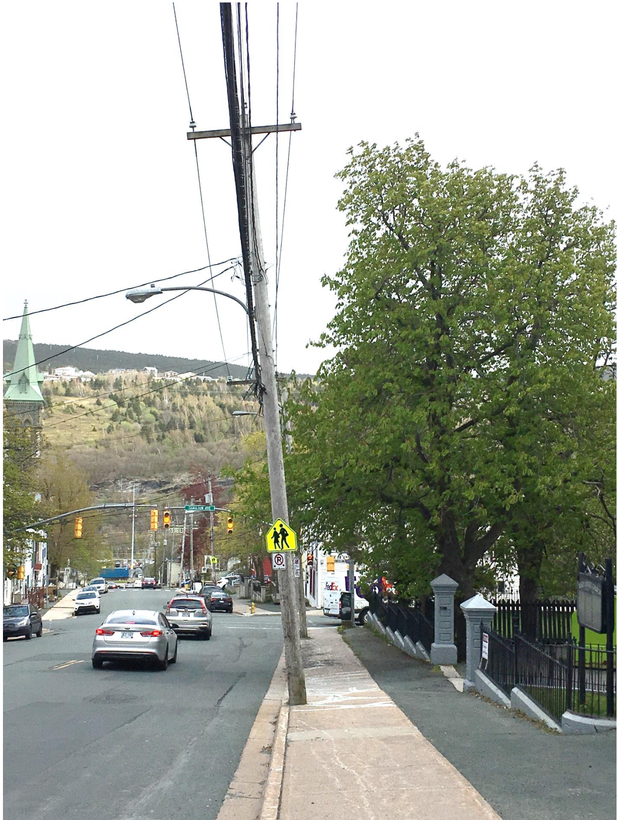
Figure 7 – Pole leaning into traffic
