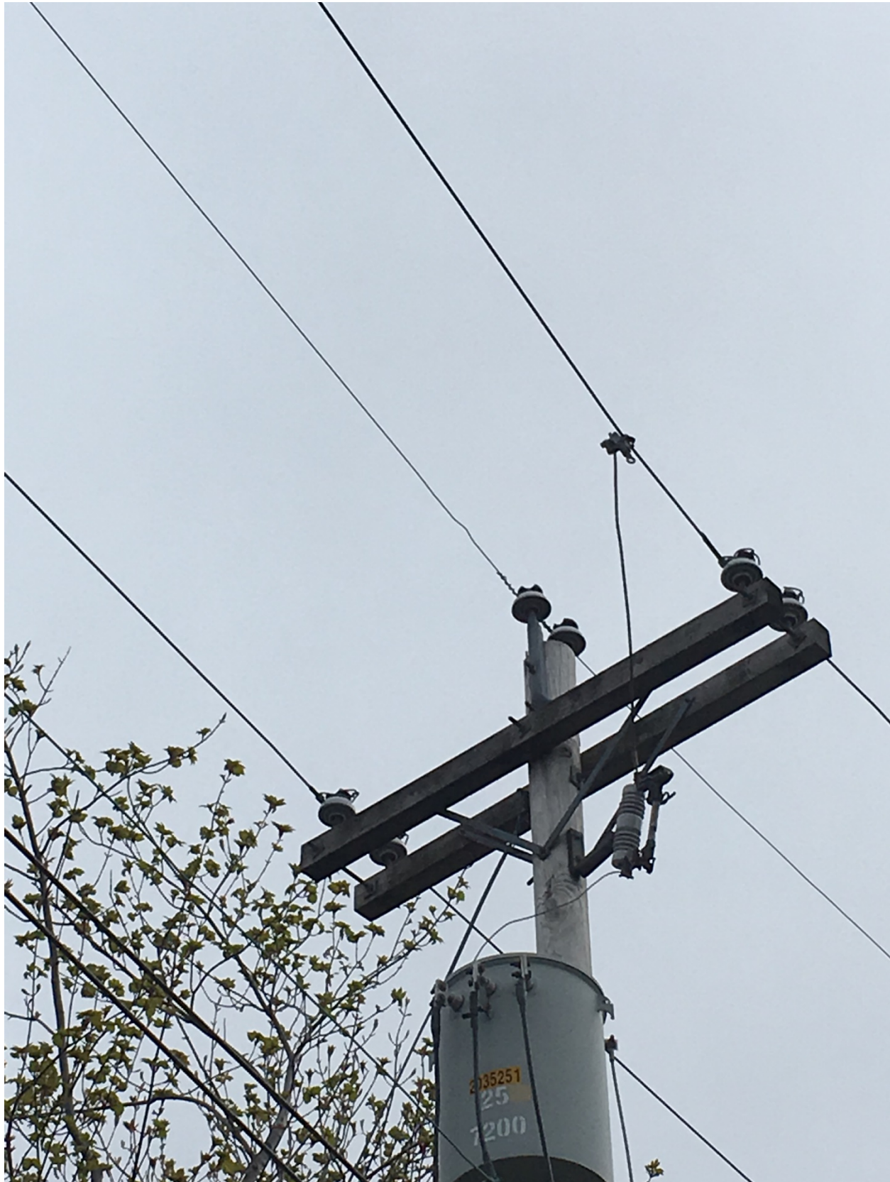
Figure 5 –#6 CU conductor
