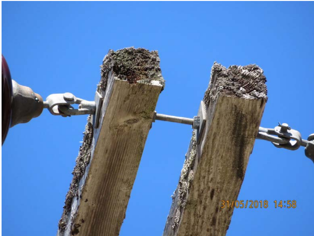
Figure 7: Cross Arm Deterioration
