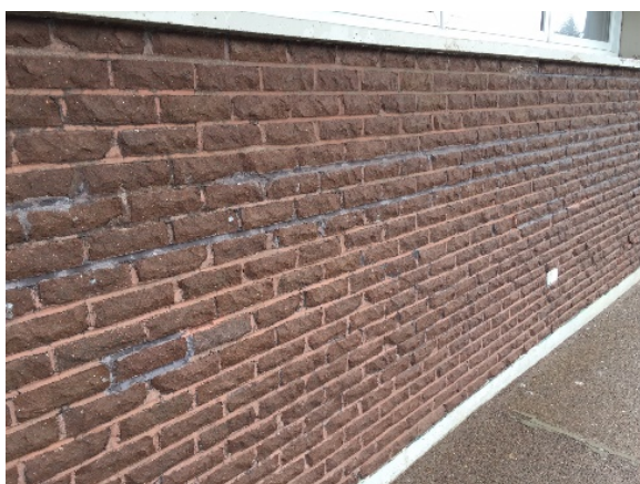
Figure 4: Re-grouted Brick
