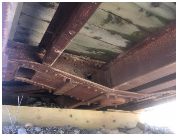
Figure 13: Temporary Abutment Repair
