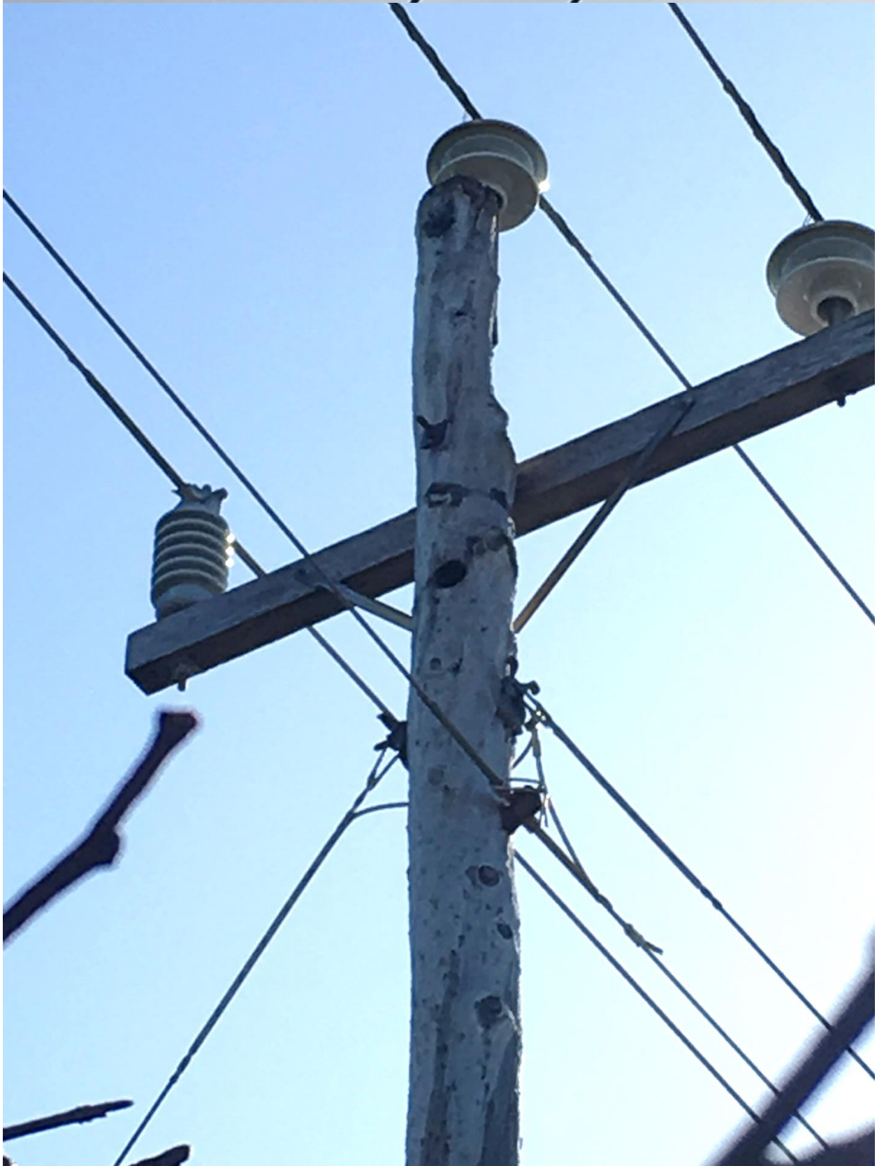
Figure 6 – Deteriorated pole. Note side phase insulator had failed previously.
