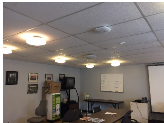
Figure 10: Incandescent Office Fixtures
