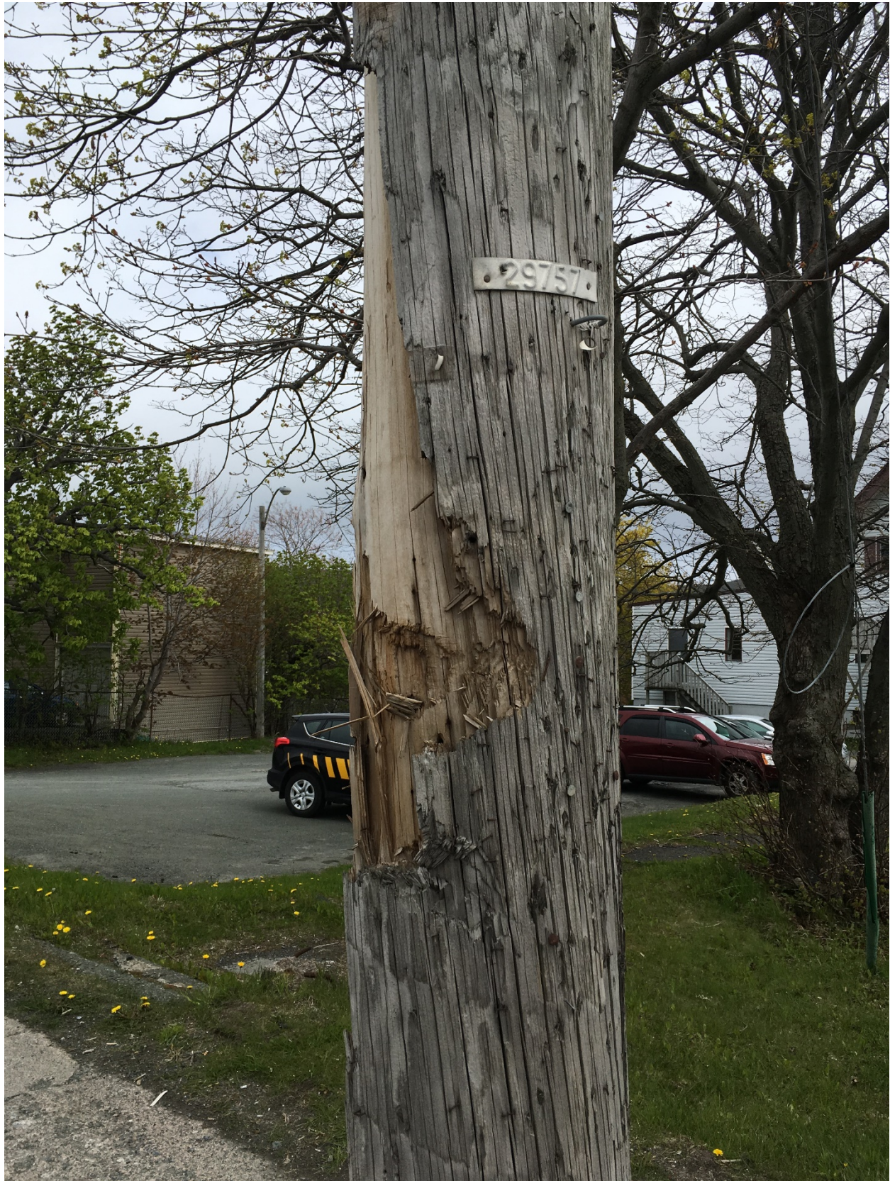
Figure 4 – Deteriorated pole with vehicular damage
