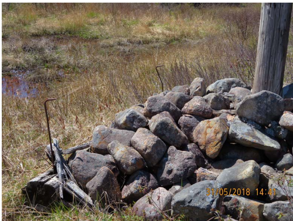
Figure 4: Rock Ballast No Longer Contained
